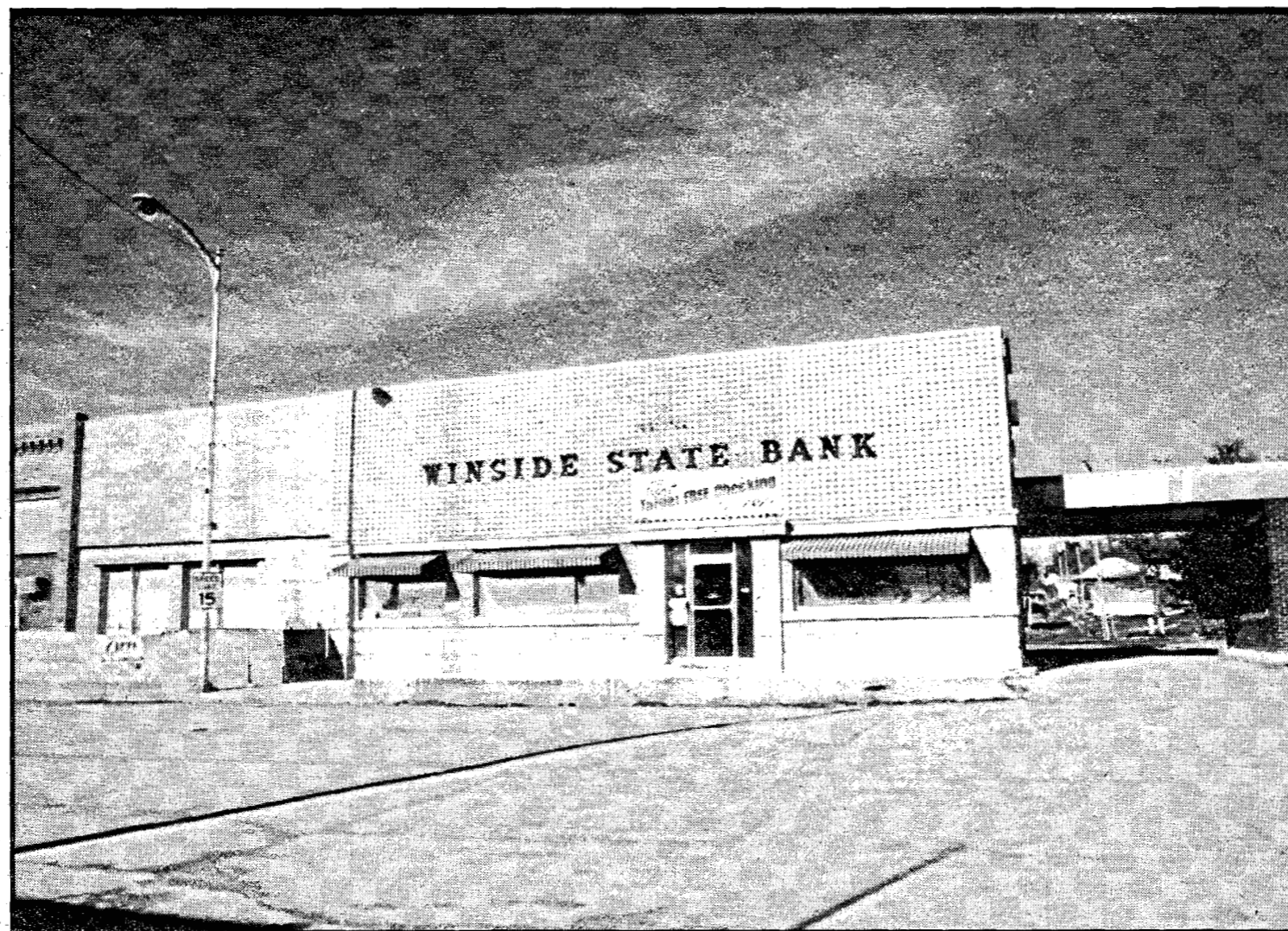
The Winside State Bank is currently undergoing a renovation which will make the building handicap accessible and create an addition on the west side of the building.
